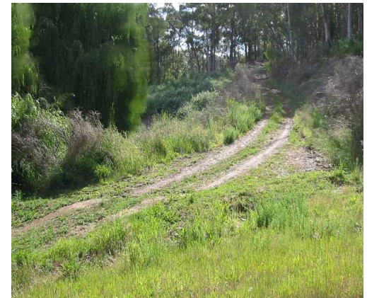
This well constructed track has been shaped with a wide, grassed drain (right of track) to transport water, and a cross drain (foreground) to carry water safely over the track. It has been surfaced with rubble and is well compacted
